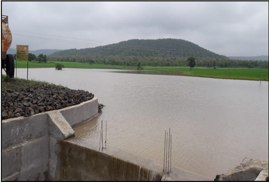
Earthen Dam Village Gundai Storage Capacity 2600 cum
