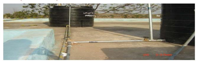
Mixing of water by dilution technology to provide 32mm GI pipe for rain water and 15mm GI pipe for fluoride water and mix in a point to provide a T socket or a small chamber(75% rain water&25% fluoride contaminated water) as permissible limit. Two regulatory valve has been provided on both GI pipe for the regulation of water, if required in future to change the ratio of water quantity from both
